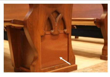
velocity supply system to use the natural effects of heat rising to provide efficient comfort.
